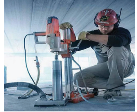
Core sampling to detect chemical contamination in concrete flooring
